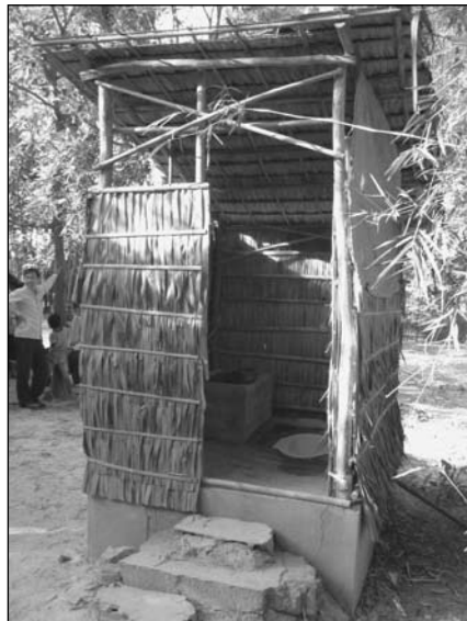
Installed Easy Latrine with palm leaf superstructure
